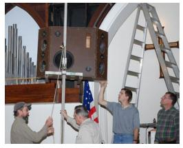
A total of 4 Rodgers tone cabinets, 2 on each side of the chancel, were lifted into place and a large pedal tone cabinet was installed in the existing ceiling chamber. The amplifiers for the
